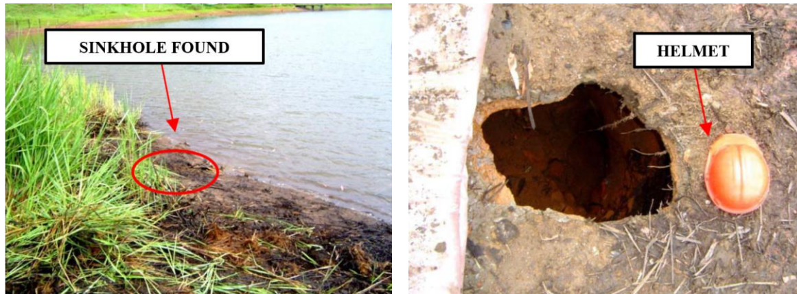
Figure 7: Location and dimension, respectively, of the sinkhole found in the upstream slope of the Gegraf dam
