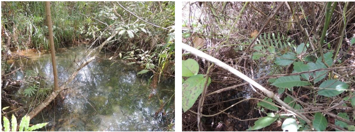
Figure 5: Water accumulation at the toe of the dam
