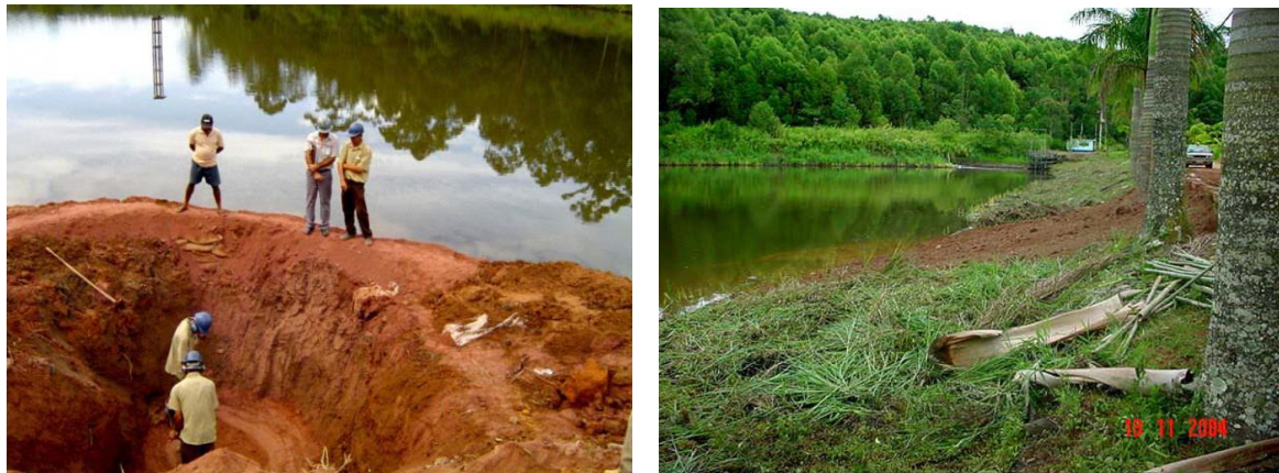
Figure 8: Compaction of clay material and protection of the affected site with organic soil
